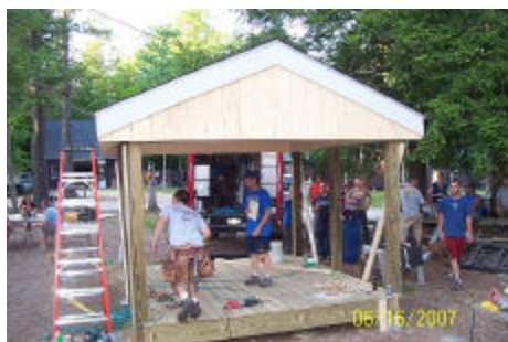
Rick discussing construction with Tony
