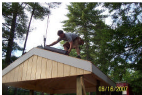
Tony working on the pavillion's roof
